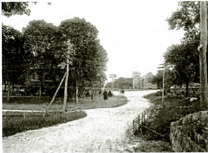
The Crossways, in the trees at left; BCC in the distance; stone retaining wall where it is today. Photo ca 1900
